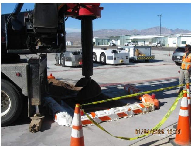
Auger base hole at hold room
