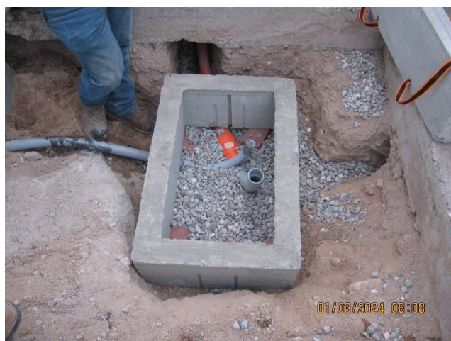
Pull box installed
