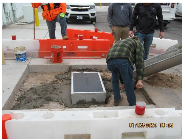
CLSM backfill at Service #1
