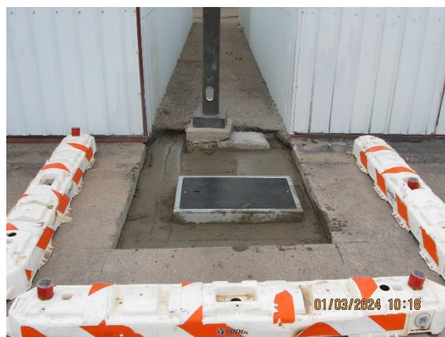
CLSM backfill at service #2
