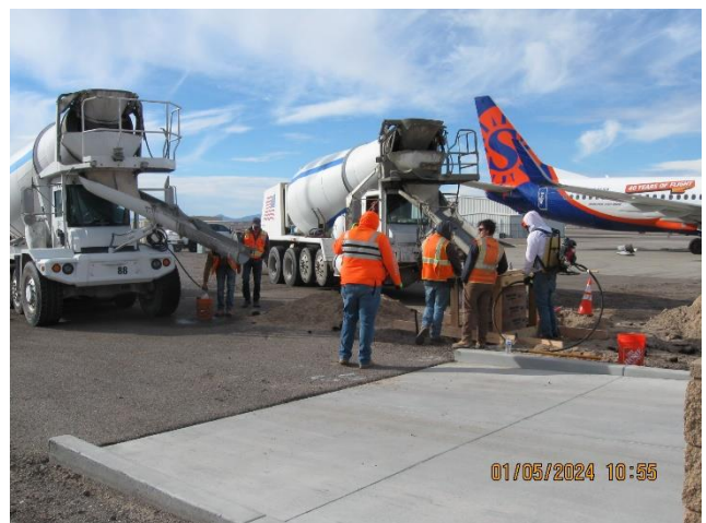
CLSM backfill and Concrete placement
